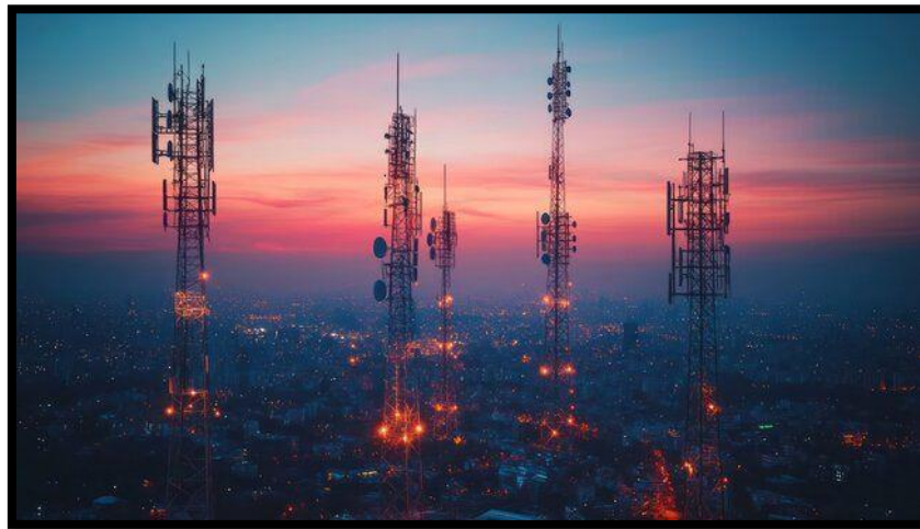
5G network antennas
